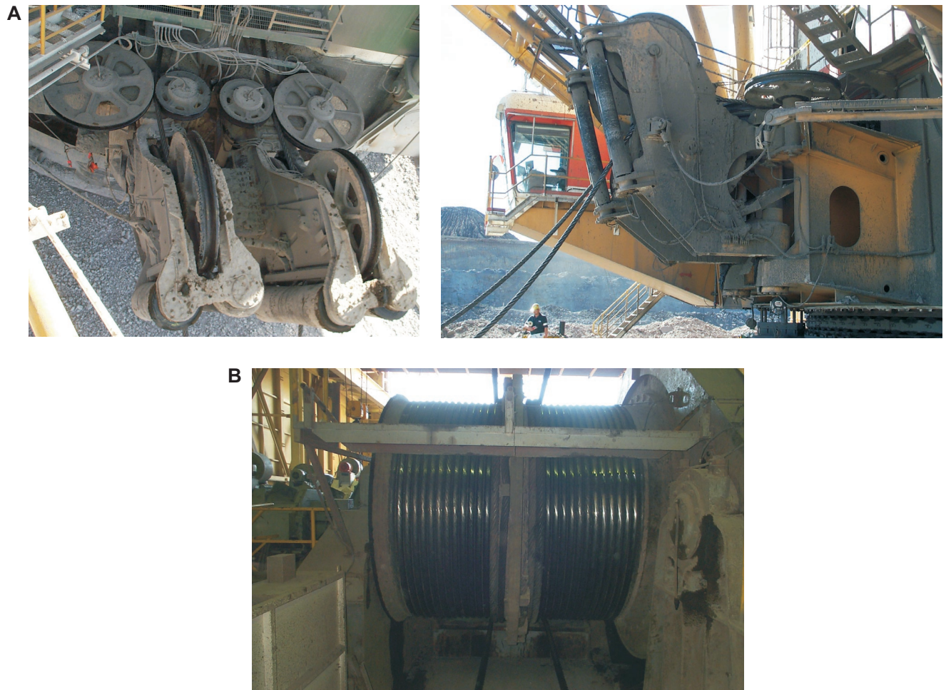
FIG 2 - BE dragline accessories for drag ropes. (A) Lower vertical, upper vertical and horizontal fairlead sheaves, (B) drag rope drums.
