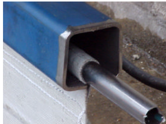
Fig 7 - Slot fixing system
