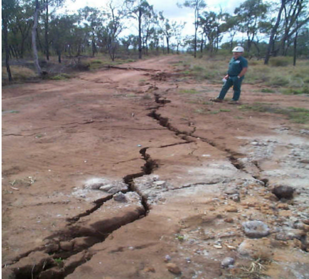
Fig 19 – Surface subsidence over fault zone – LW103
