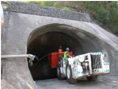
Fig 5 - Dendrobium Tunnel - June 2002
