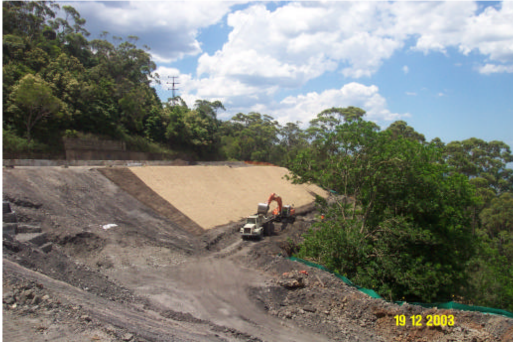
Fig 4 - Photo showing works in progress.
